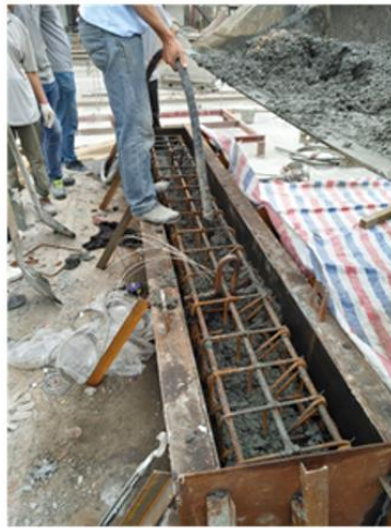
Construction of HSC Column Specimen
