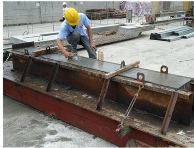
Construction of HSC Column Specimen
