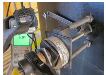
Pull-out test for anchor bolt
