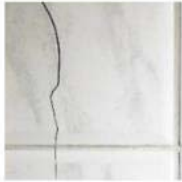
Cracks on tiles
