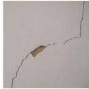
Cracks on plaster
