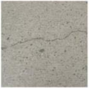
Cracks on concrete
