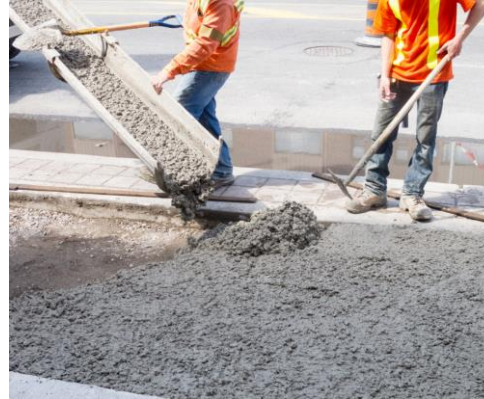
Cement and concrete curing monitoring (DTS)
